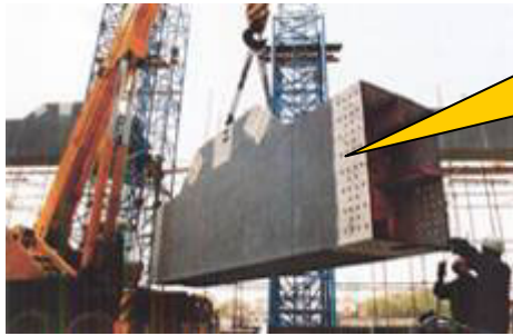
Illustration 2.3 This case was when the ditcher set up the soil-blocking steel, using the U-shape bolt, which should be fastened tightly.
