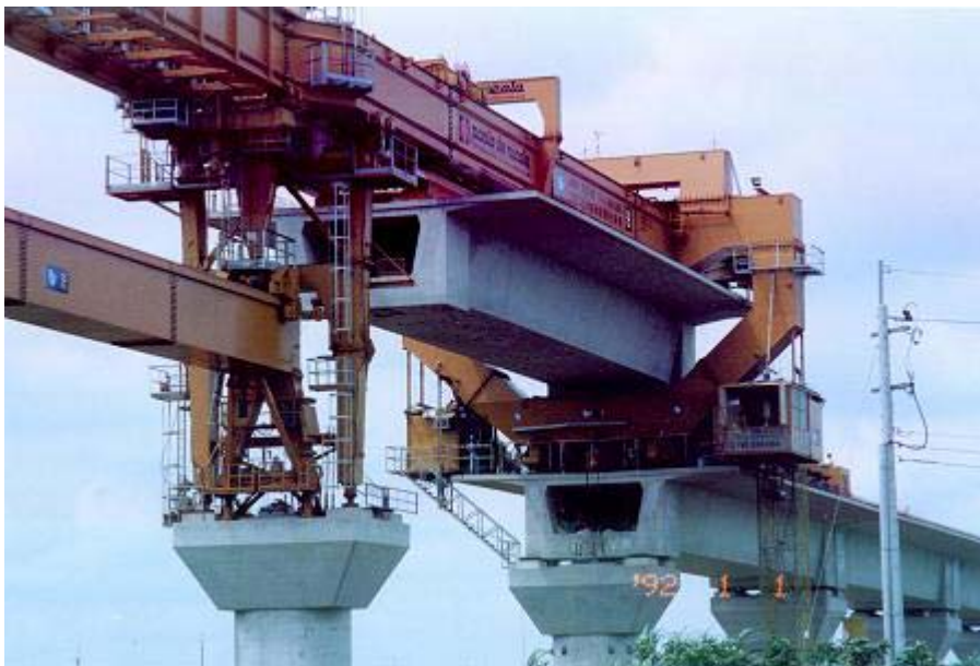
Figure 5 Pre-cast viaduct assembling
